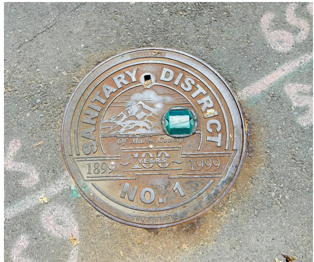
Old RVSD Manhole with Smart Cover.
