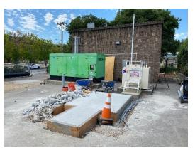
Larkspur Pump Stations 14, 24, & 25 Improvements: Construction is underway at pump station (PS) 14, which is located adjacent to Hall Middle School in Larkspur. A new photoionization odor control unit has been installed and is fully operational. The odor control unit will improve local air quality and reduce nuisance odors.
