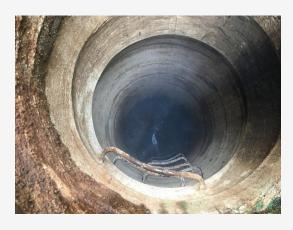
Hence, the surface area of manholes, as a potential area of I&I, is comparable to the pipes that connect them. Their rehabilitation is a central part of RVSD's efforts to keep rain water and groundwater out of the sewer system.
