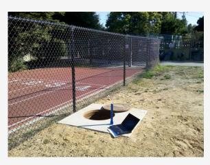
The condition assessment crew uses closed-circuit television cameras (CCTV) to continually monitor and assess the condition of the pipes and nodes (i.e., manholes, rod holes and lamp holes) in the wastewater collection system. We research and deploy the latest technology to improve the accuracy of these assessments - which are vital as they provide the foundation for our decisions about investments of time and money for capital, maintenance and repair programs.
