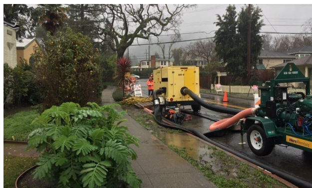
Bypass pumping during a storm
