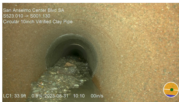
CCTV footage of the 10-inch pipe clogged with gravel
