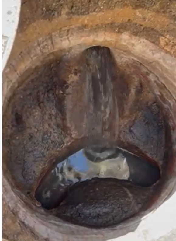
Diane Lane manhole with unpermitted Force Main discharge
