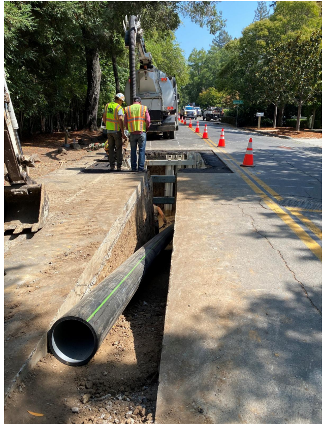
Precision Engineering installing new 12-inch sanitary sewer main on Woodland Road
