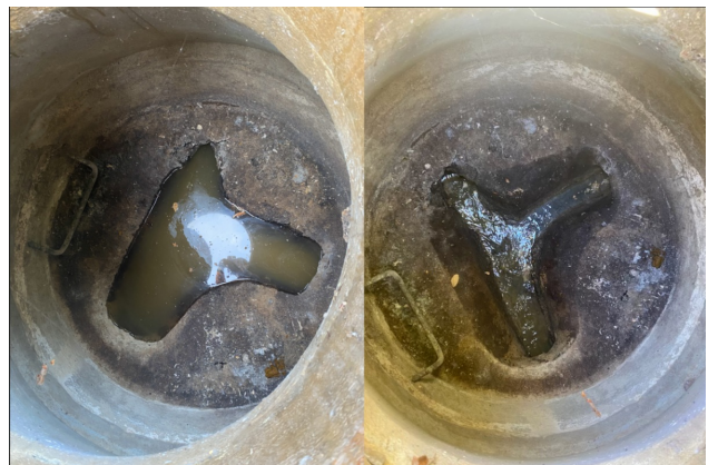
Surcharged manhole before and after.
