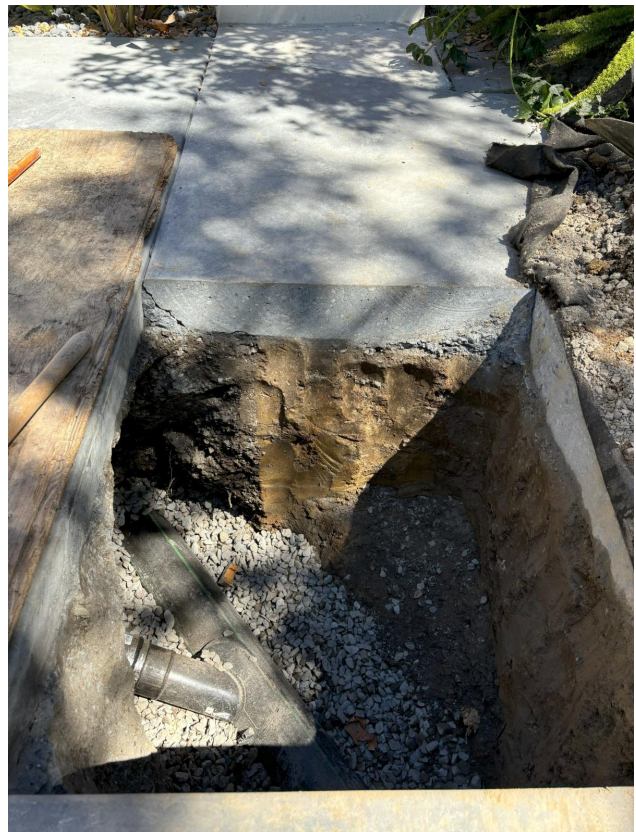
Driveway Lateral Connection in Greenbrae
