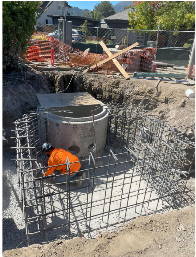
Pump Station 31 Valve Vault Construction
