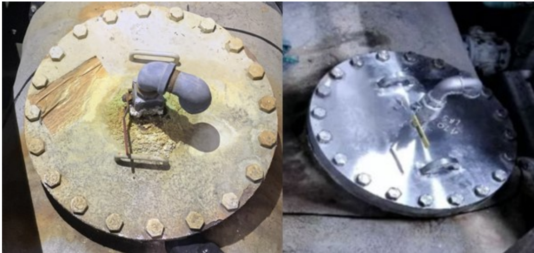
Before and After: Replacement of the Rusted 2-Foot Blind Flange
