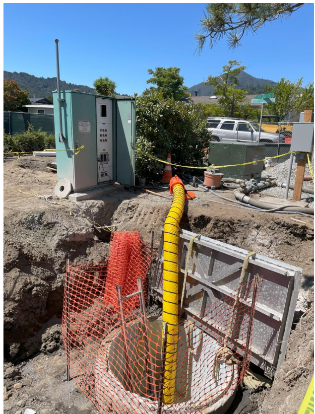
Pump Station 32 Wet Well Installation
