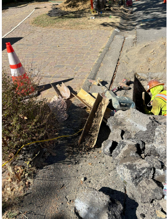
Removing Old Pipe
