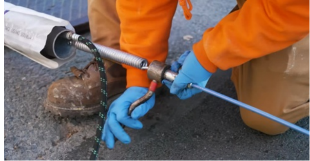
Staff preparing a trenchless point repair
