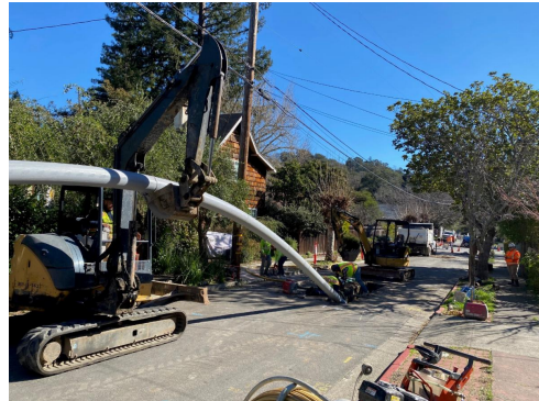
Construction crew working on a sewer replacement.
