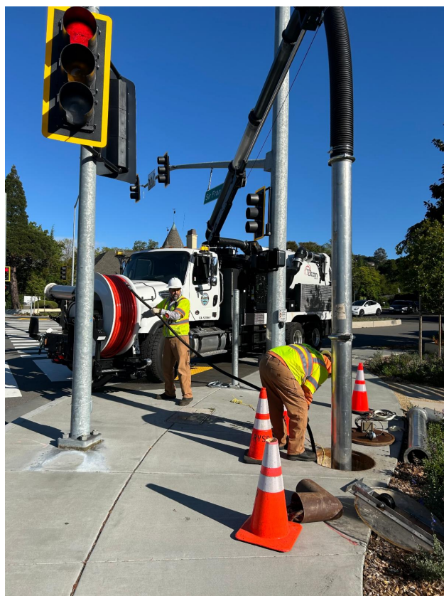
Staff cleaning 10-inch lines on Sir Francis Drake Blvd in Greenbrae.
