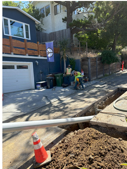
Replacing 100-year-old sewer line and laterals in Fairfax.
