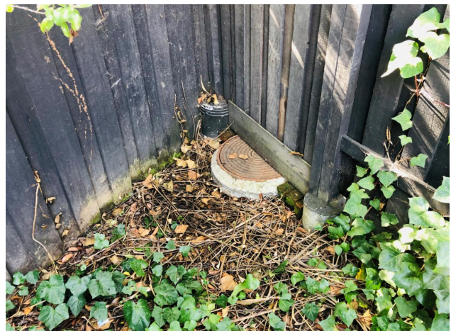
Fence Built on Manhole.
