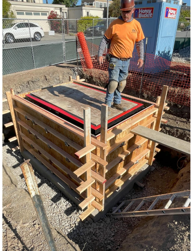
Construction of Flow Meter Vault
