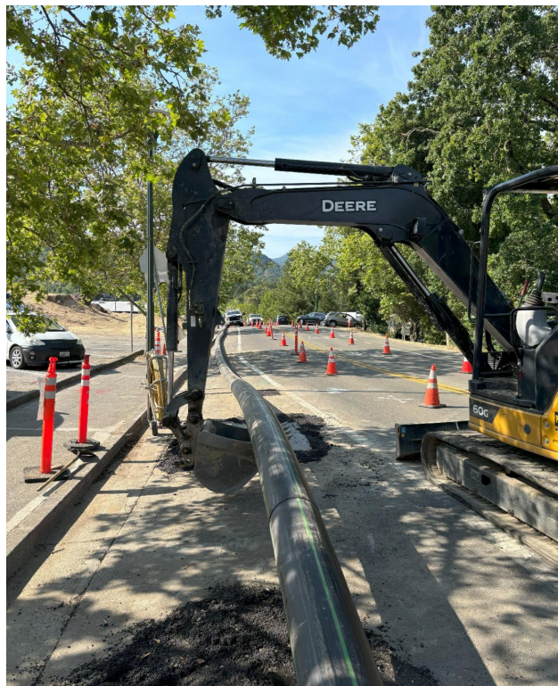
Replacing Old Sewer Main in Fairfax
