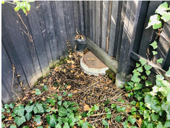
Fence Obstructing Manhole
