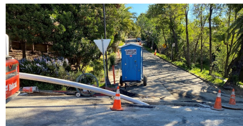
FY 23/24 Gravity Sewer Improvements Project Pipe Bursting
