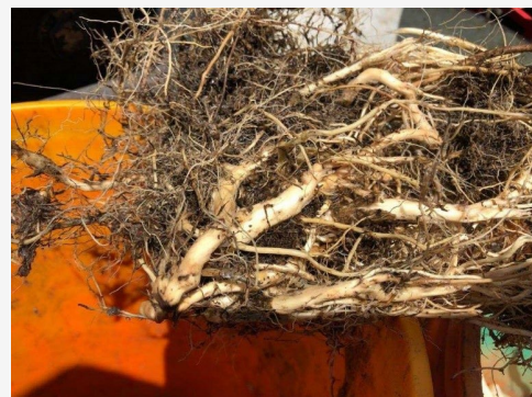
Tap root mass removed from sewer using hybrid nozzle
