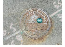
it's a SmartCover. Staff responded to a SmartCover high-level alarm located at a manhole in Larkspur on Diane Ln. Upon arrival, Staff observed the sewer main backing up. Staff relieved a soft blockage 69 feet downstream using a high-pressure flusher.
