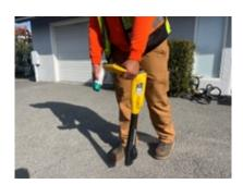
Due to traffic and hospital infrastructure, this specific bypass force main has been challenging to locate. To find the pipe, staff had to temporarily shut down PS 25 at 1350 South Eliseo Drive so that a locating rod could be inserted in the pipe. The rod emits an electromagnetic signal that allows staff to locate the underground pipe using a locator wand. While locating, staff periodically mark the asphalt with spray paint to show the pipe's location.
