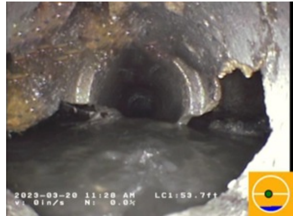
Example of a void in a clay sewer pipe.
