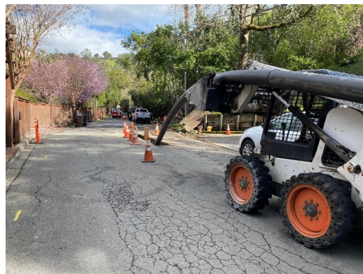
Glosage installing new HDPE pipe
