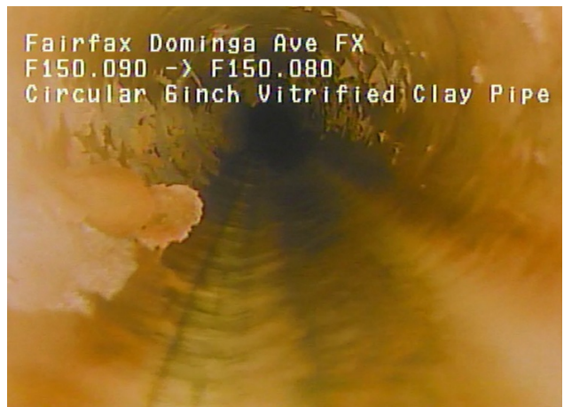
CCTV footage of the Dominga Ave clay sewer pipe.
