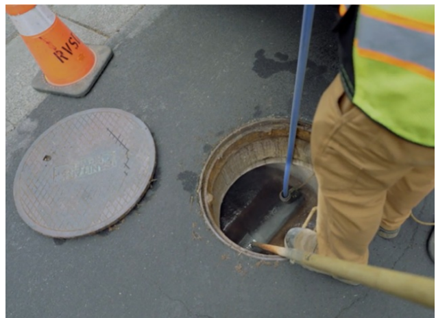
Line Maintenance cleaning a sewer pipe with a high-pressure water hose.
