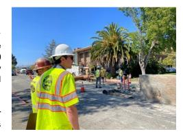
throughout the District service area. Improvements include upsizing a 6-inch sewer line to an 8-inch line to increase system capacity on The Alameda (San Anselmo) where a sanitary sewer overflow occurred last year.
