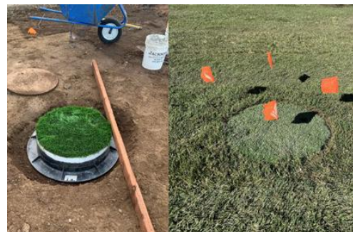
Construction of the turf manhole
