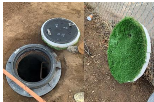
Construction of the turf manhole
