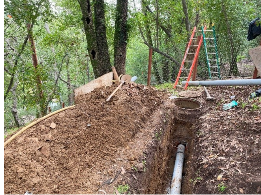
Gravity sewer replacement in an easement.
