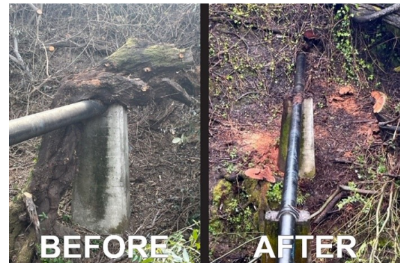
Before and after of the creek crossing sewer main.
