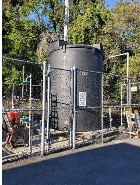
Nitrate tank outside Pump Station 13
