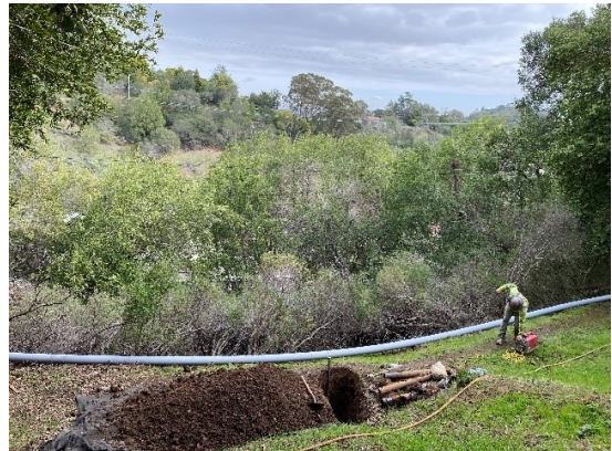
Glosage installing a new sewer main in the Vista Grande Easement
