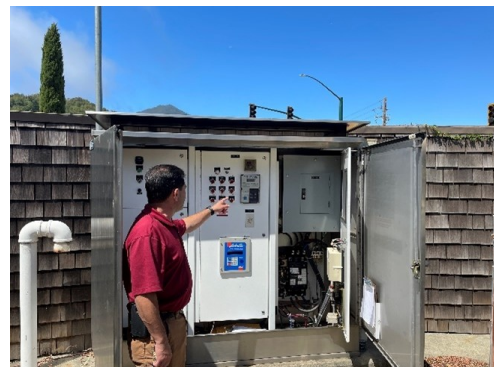
Noel Sandoval, the Pump Station Crew Supervisor, showing a Pump Station 25 Alarm Panel
