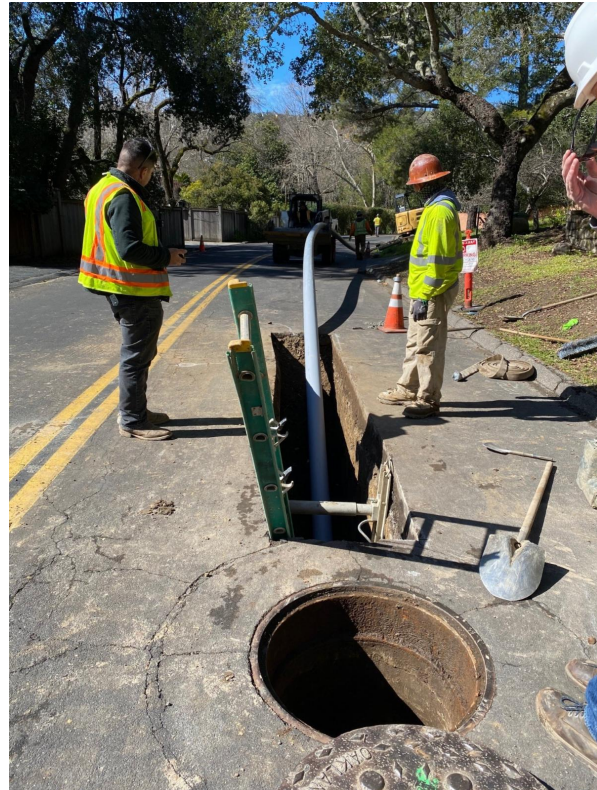
Construction crew working on a sewer replacement.
