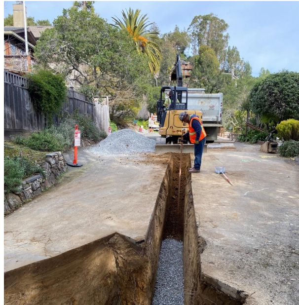
Open-cut installation
