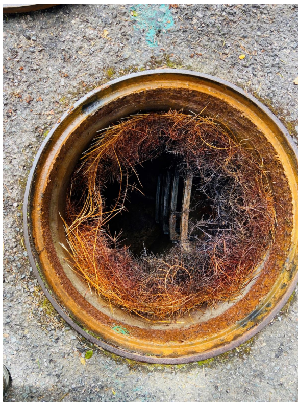
Roots invading a manhole
