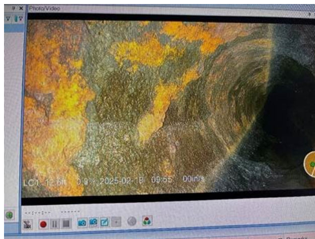
Corroded steel on crown of FM14, twelve feet upstream of leak location
