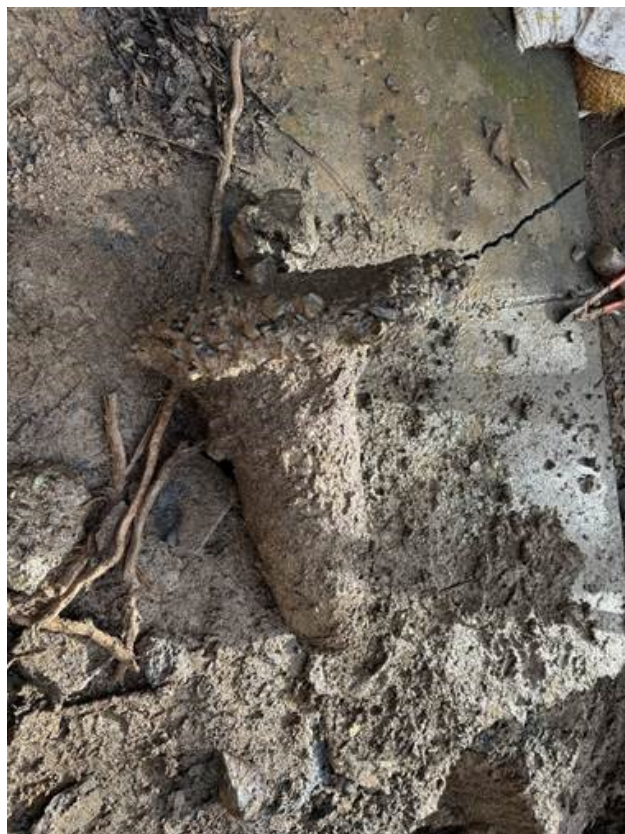
Fence posthole concrete that was poured directly onto the FM14 pipe where it spilled
