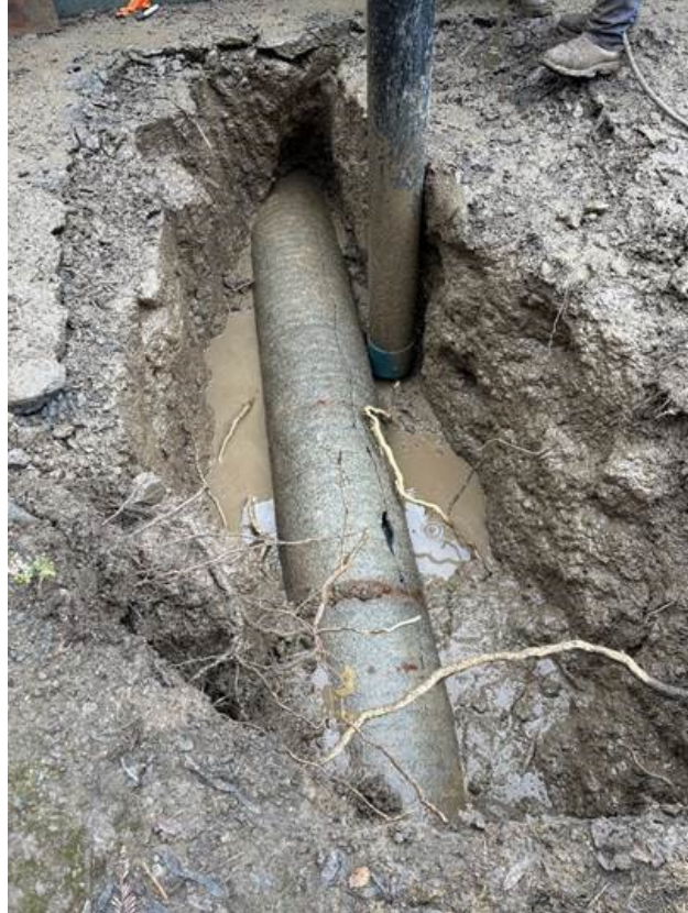
FM14 pipe defects at location of leak
