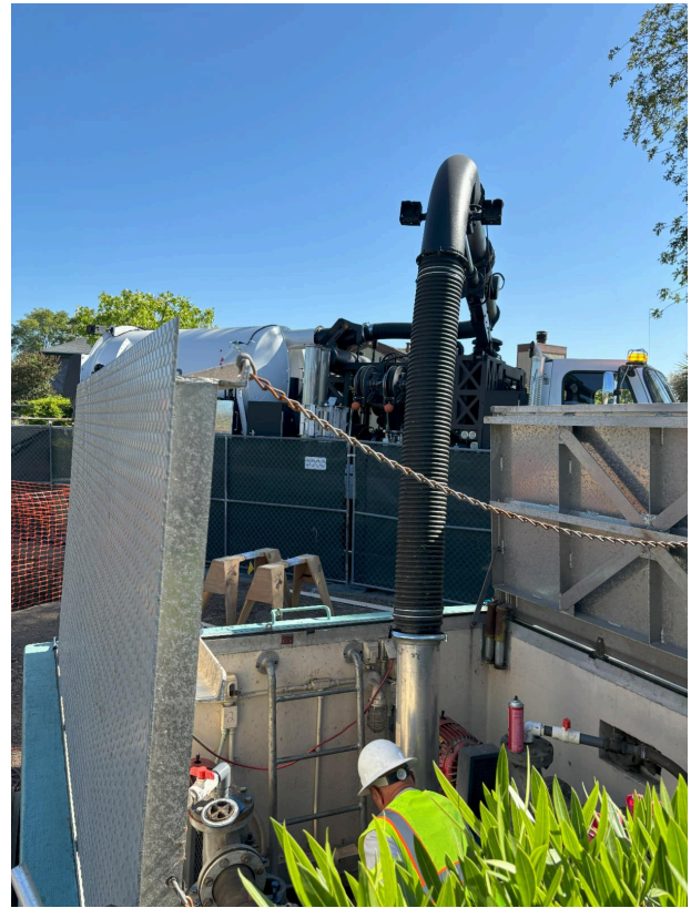
Wet Well Cleaning in Progress.
