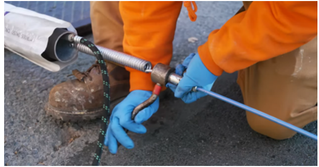
Staff Preparing a Trenchless Point Repair.
