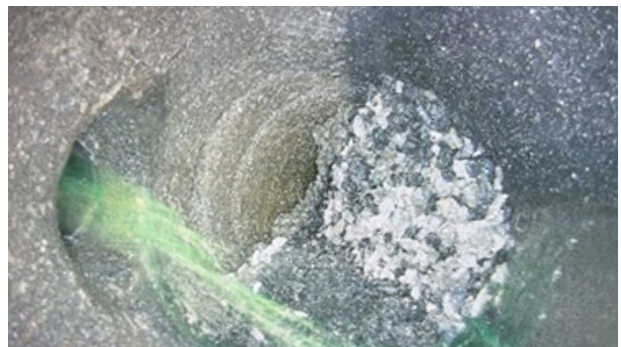
Dye Test of Public Sewer Containing 3/4-Inch Rock Debris.
