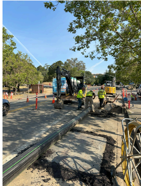
Replacing Old Sewer Line in Fairfax.
