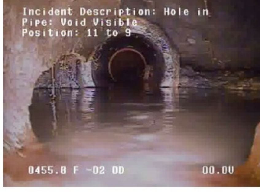
Grade 5 defect showing a visible hole in pipe
