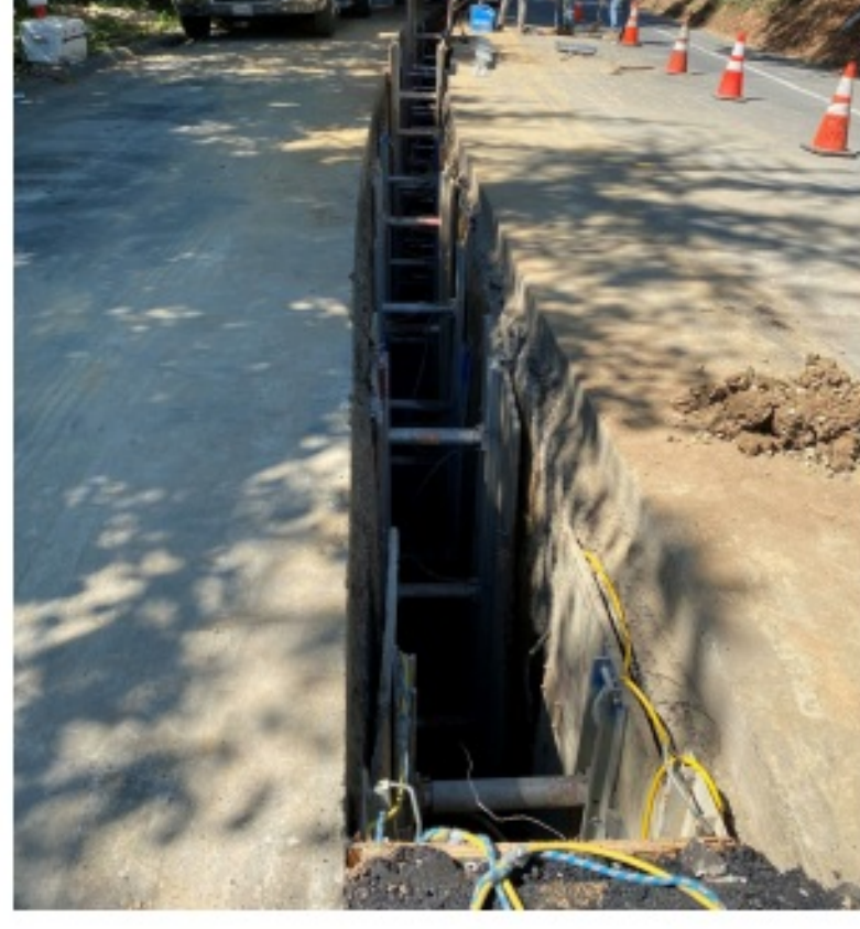
Open trench excavation for pipe installation
