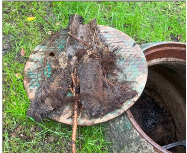
This tree root was growing through a manhole.
